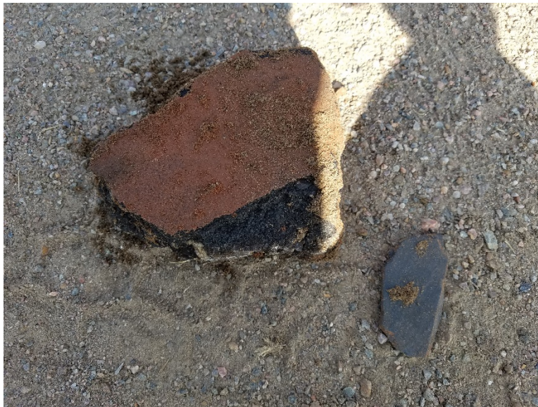
ACM Mastic on Brick
