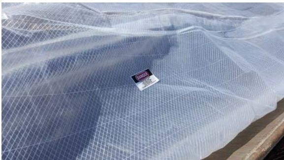
Wrapped load with asbestos hazard labeling.
