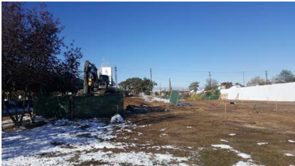
Beginning of excavation of mound at grid 2D.
