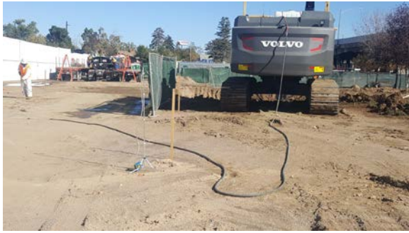
Water hose attached to excavator for continuous operation of water sprayer.
