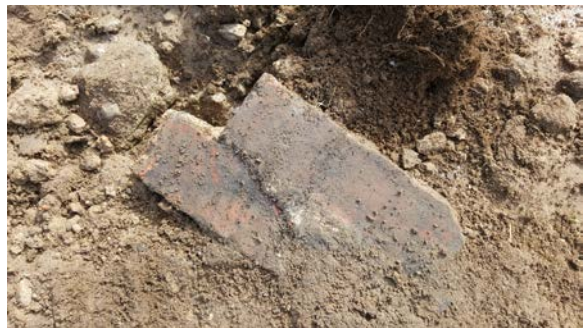
Debris - brick with mastic.
