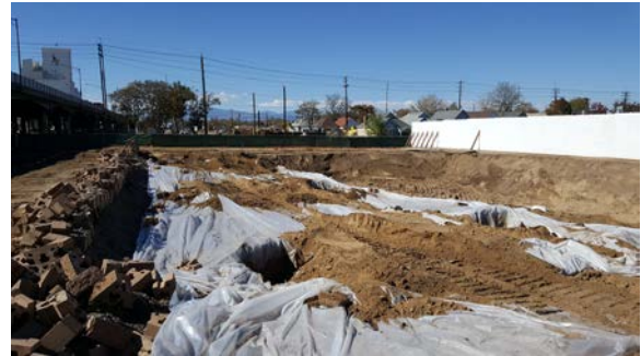
Potholes were dug to 10 feet and then filled back in. No debris was found except for a metal rod.
