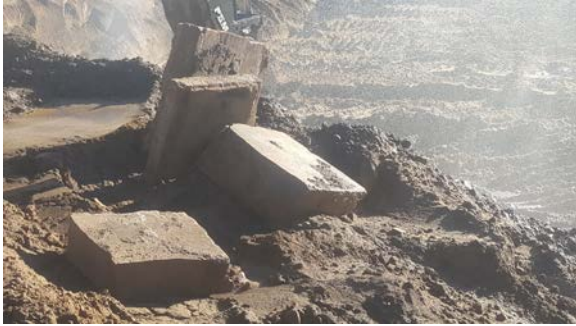
Concrete foundation found in grid 5A and west of 5A.
