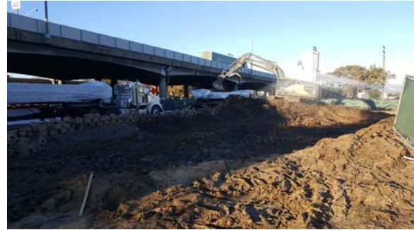
Start of work on day 2, west end of mound.
