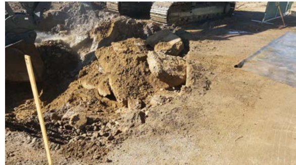
Concrete foundation encountered in grid 2B.
