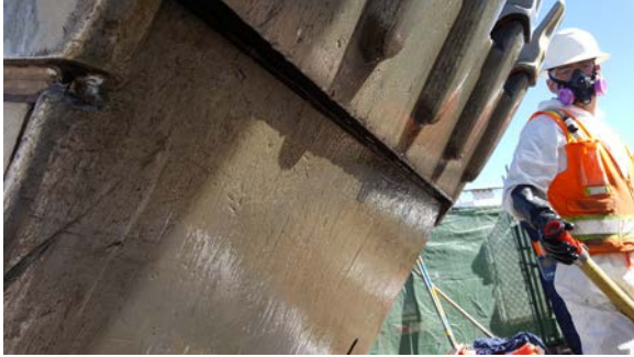
Bucket was then cleaned with low pressure water, which was collected in a basin for filtration.
