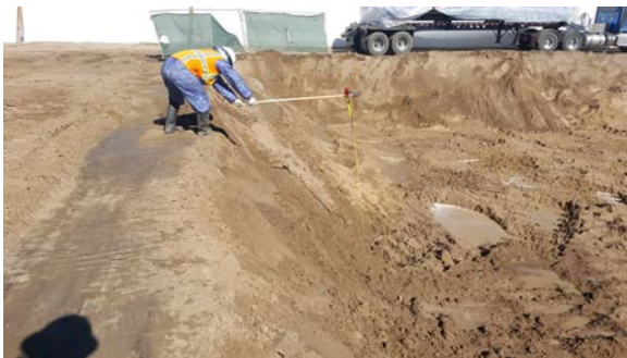
Confirming depth of 8 feet on west side of excavation.
