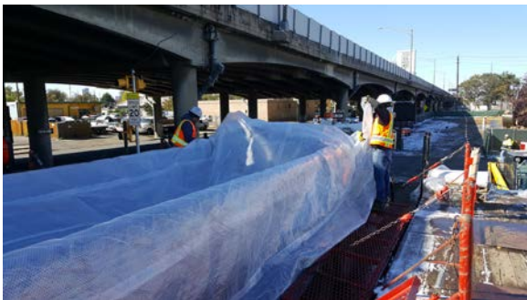
Truck wrapping station. Workers placed two layers of reinforced polyethylene sheeting.
