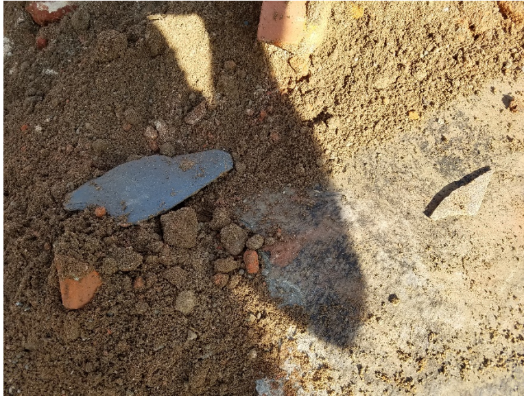
ACM Mastic on Concrete and ACM Floor Tiles
