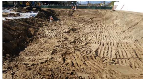
No debris remained in the excavated area.
