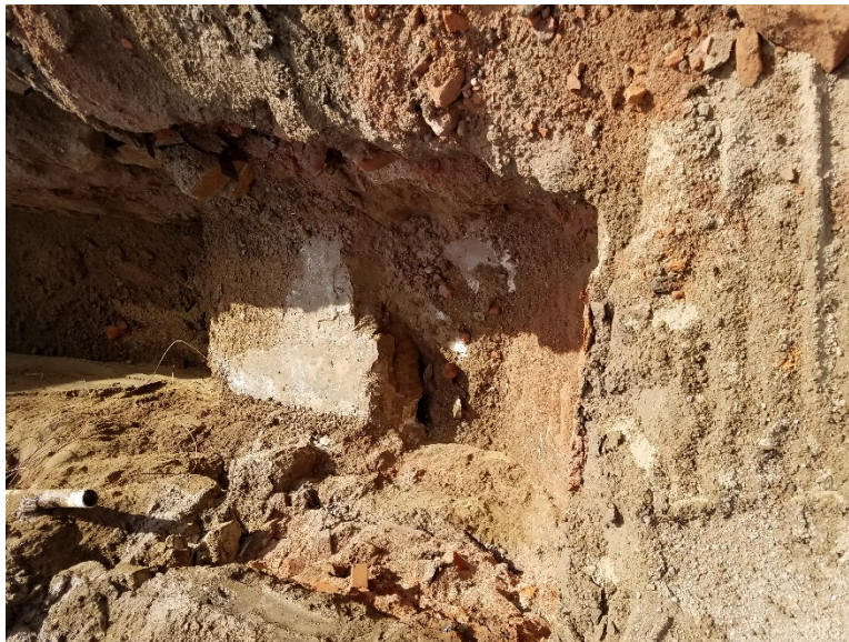
Building Footer found in Grid 2B
